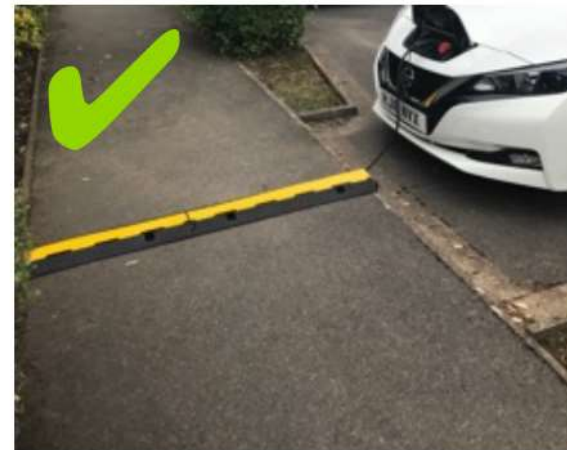
Figure 30: Guidance for laying of EV charging cables across a footway
